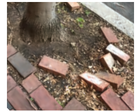
Have your loose bricks reset and leveled.
